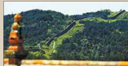
Ancient walls in Chengde
